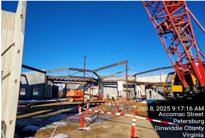
Structural Framing For Max Units
