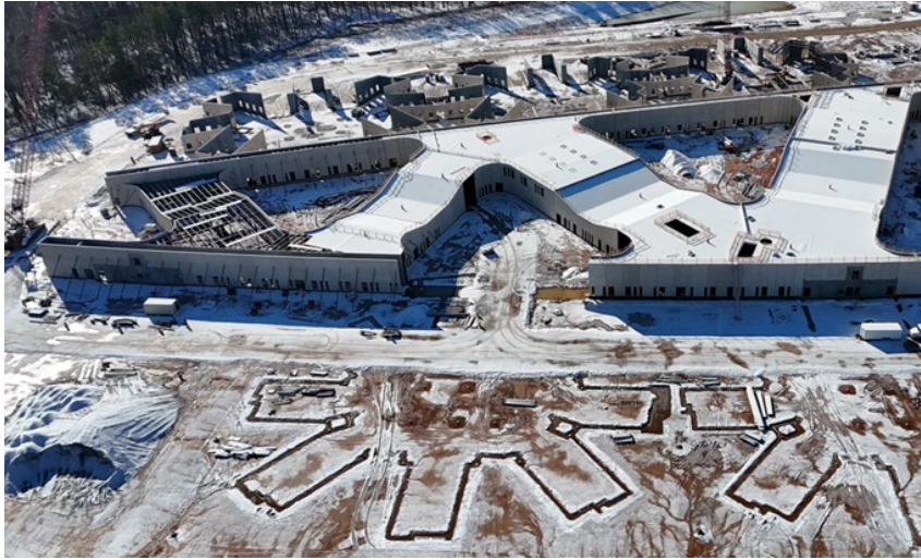
Treatment Mall structural framing
