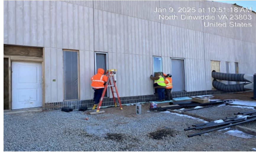
Installing windows in exterior walls
